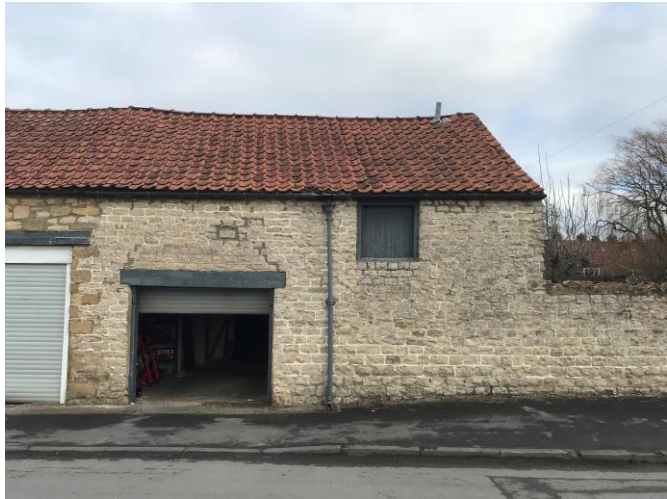
Pic 1 – View looking north on the primary façade of the barn. Historic openings visible.
