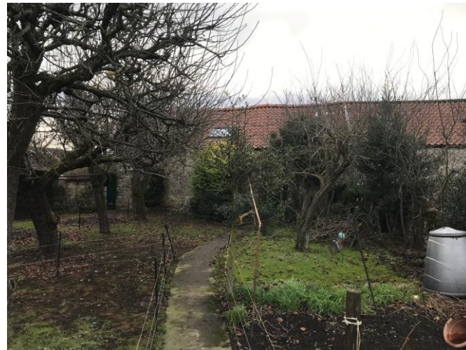
Pic 4 - View looking south onto the northern façade. The building is generally hidden by mature planting and trees.
