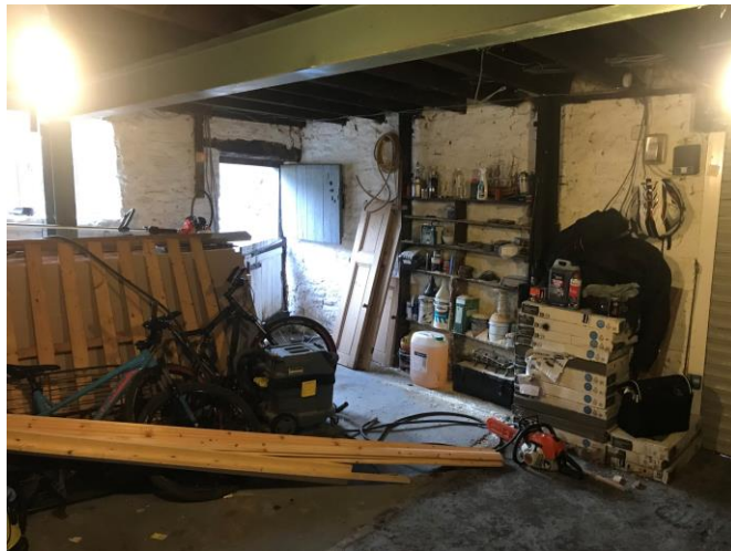
Pic 11 – Internal view of ground floor workshop area.
