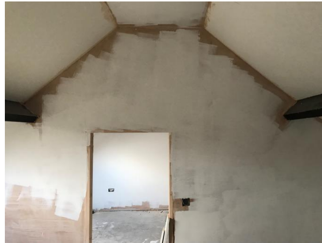
Pic 10 – Internal view of first floor – all areas boarded out.
