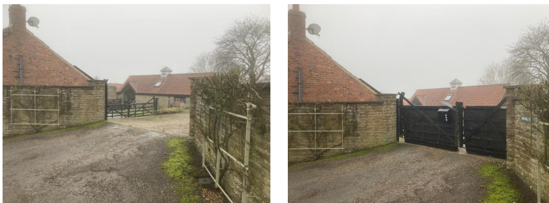
d) View of S courtyard from N Back Lane
