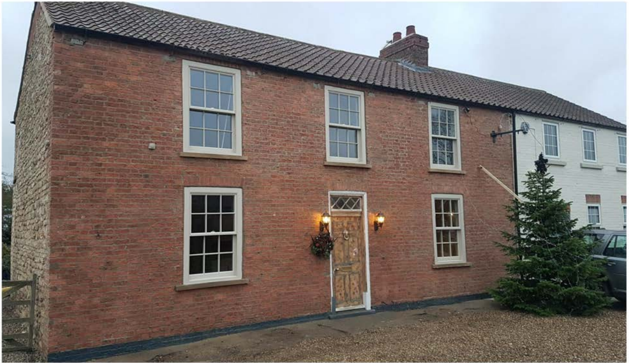
THE WHITE SWAN INN, LOW STREET, THORNTON-LE-CLAY, YO60 7TG
